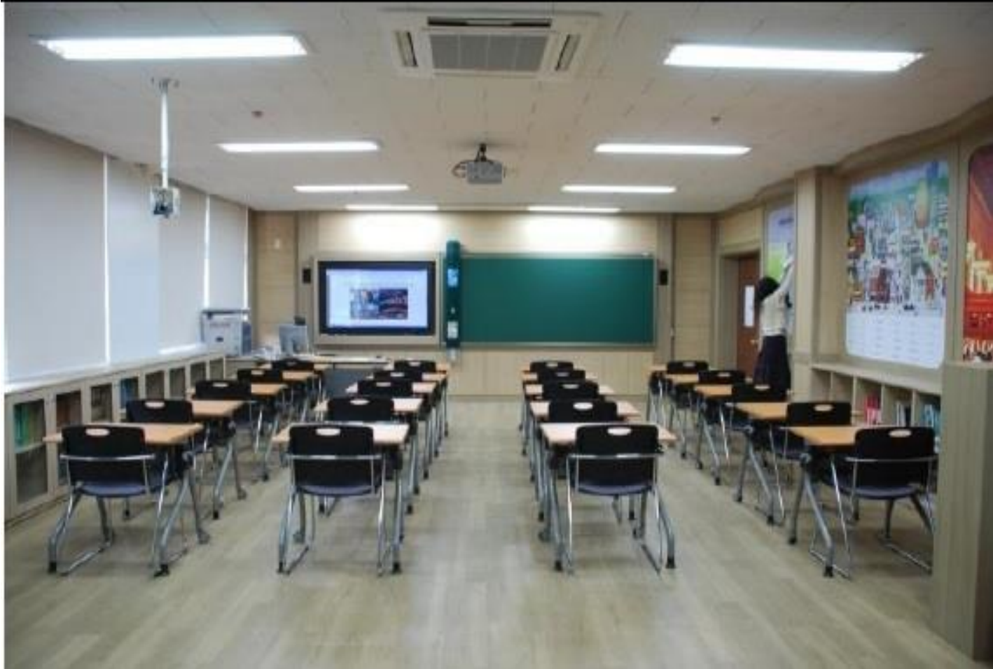
Lighting in a Smart Classroom
